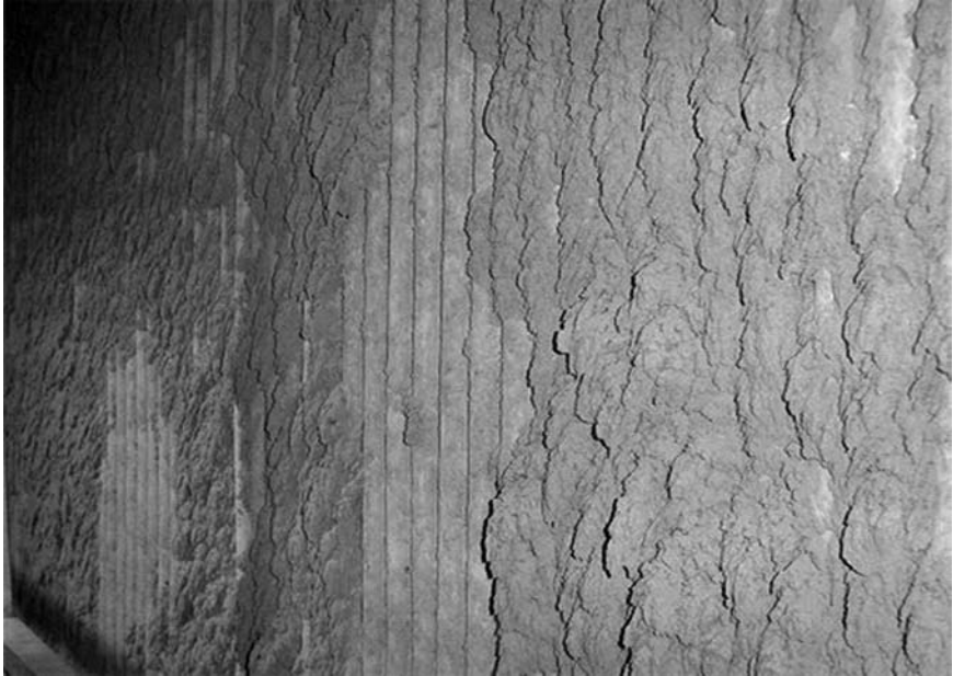
Figure 24: Example of fouled water tube furnace wall [23].
