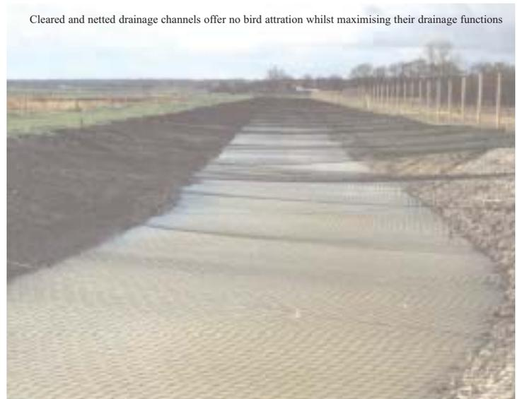
Cleared and netted drainage channels offer no bird attraction whilst maximising their drainage functions
