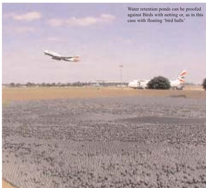
Water retention ponds can be proofed against Birds with netting or, as in this case with floating 'bird balls'
