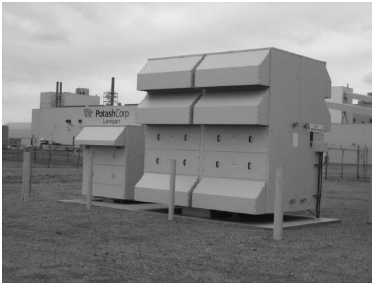
FIGURE 3.5 Outdoor three-phase dry-type resibloc transformer. (Courtesy of ABB.)
