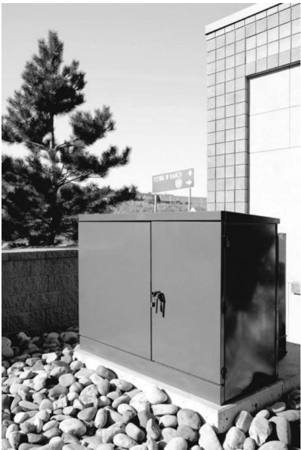
FIGURE 3.11 Pad-mount installation of three-phase resibloc transformer. (Courtesy of ABB.)
