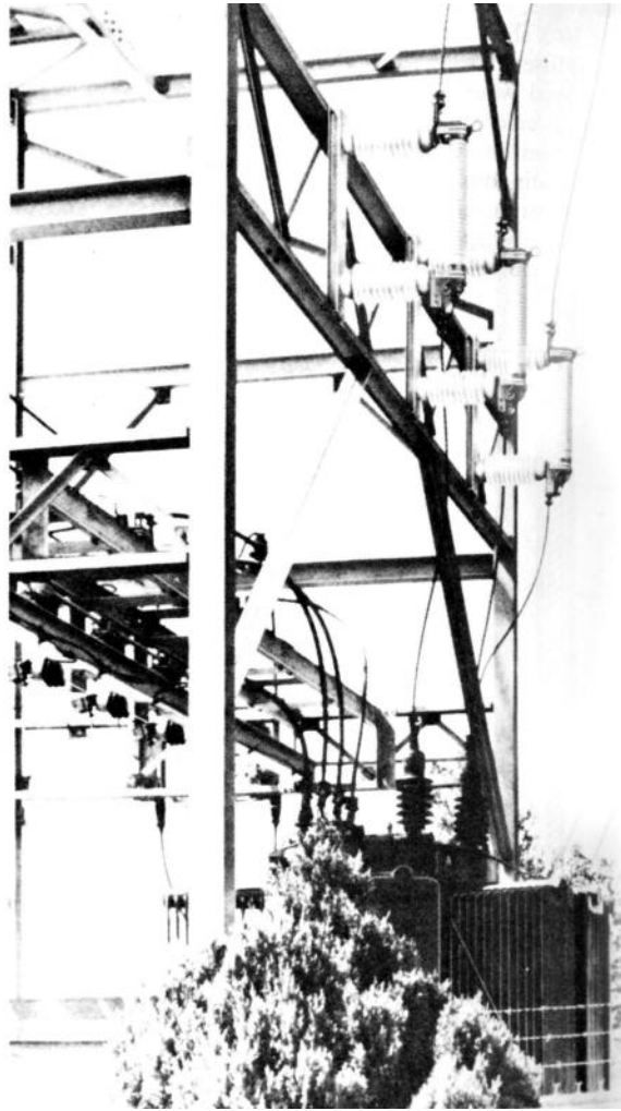
FIGURE 10.6 Typical transformer protection application of 34.5 kV SM-type power fuses. (Courtesy of S&C Electric Company, Chicago, IL.)
