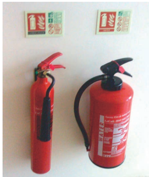
Figure 1.44 CO 2 and water extinguishers and information posters
