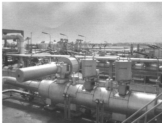
Figure 18.38 One ball valve for ESD and two axial on-off valves for HIPPS Courtesy of Mokveld Valves BV
