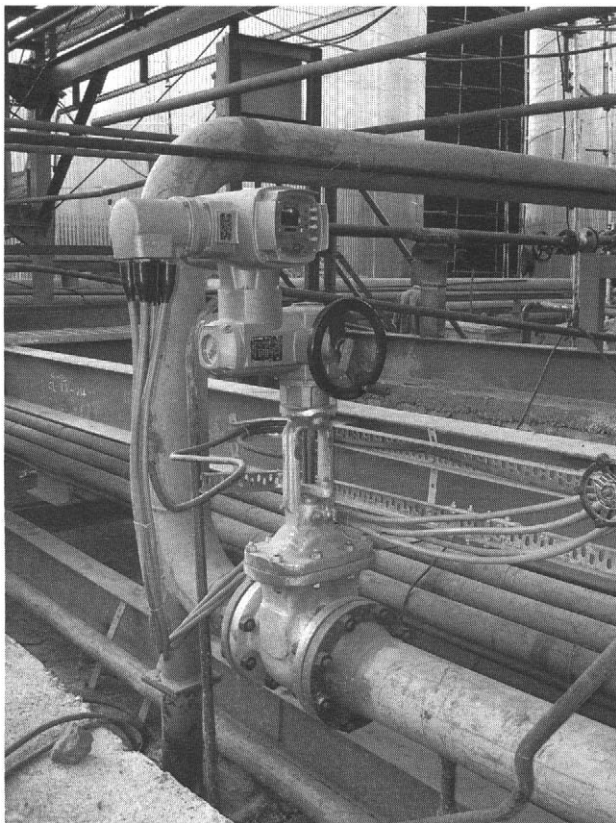
Figure 18.20 Electric actuators in a flow control application Courtesy of AUMA Riester GmbH & Co KG
