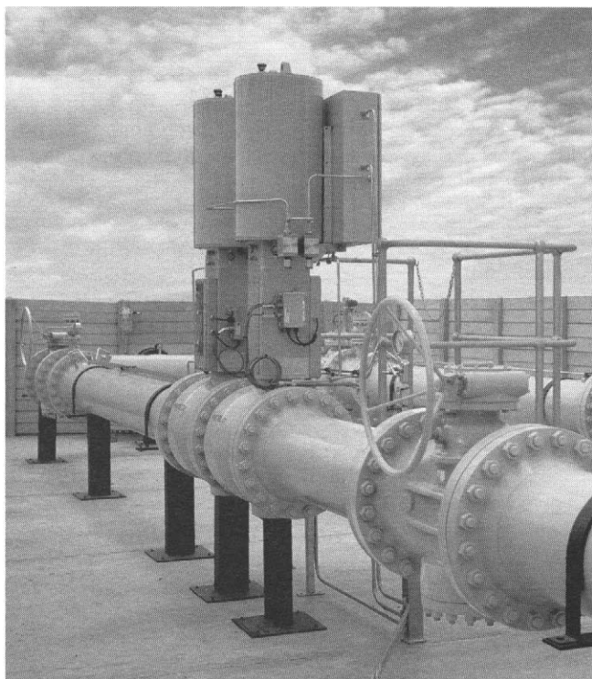
Figure 18.37 Control and safety system consisting of an axial control valve and axial isolation HIPPS valve according to IEC 61508
