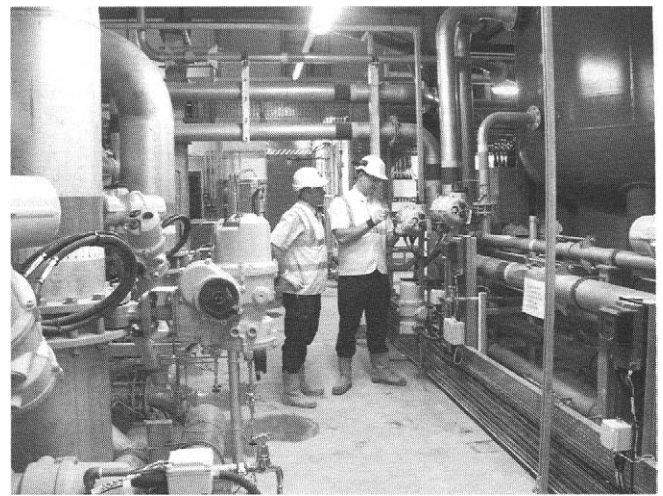
Figure 18.53 Uploading commissioning data on an actuator installed in a UK water filtration plant
