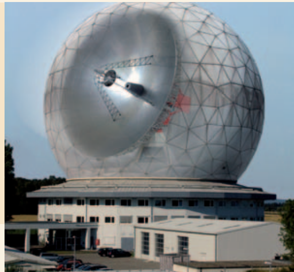
The Fraunhofer-Gesellschaft analyses space debris using the space observation radar system TIRA as well as other space objects, thereby contributing to safety in space.
