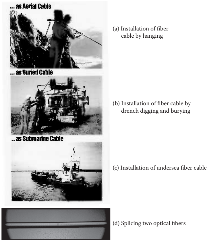
FIGURE 6.18 Installation of fiber cables at different terrains and undersea.
