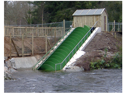
Figure 2.9 An example of an Archimedian screw at the River Dart country park, Devon. Credit: WRE Limited.
