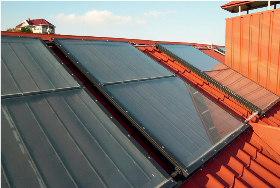
Figure 2.3 Photo of a solar hot water panel.
